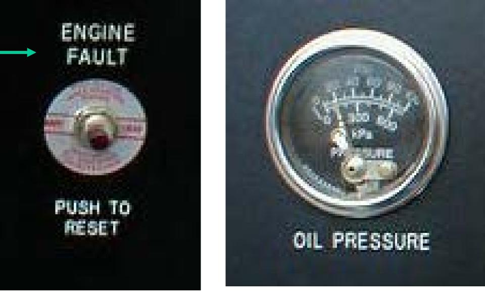
You must push this button in and then watch oil pressure gauge until it goes up past switch setting
