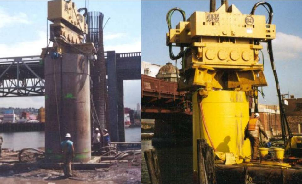
A vibro is a tool that, when attached to a pile, shakes it up and down in a vertical motion for the purpose of installing or removing attached to a pile.
